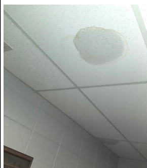
Ceiling leaks in the men’s bathroom
