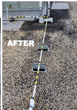
Rooftop HVAC gas pipes insulated and protected
