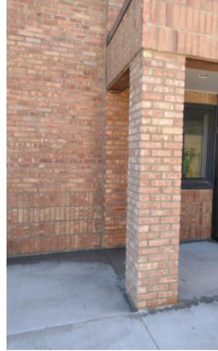
**Parish Work from last week:** due to structural damage, the pillar on the north side of the parish office was entirely rebuild and the entire wall was pressure washed to clean black streaks and water proofer was applied to prevent future build up. Job cost \$4,400.
